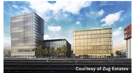
Courtesy of Zug Estates University of Applied Sciences and Arts, School of Information Technology, Campus Zug-Rotkreuz
